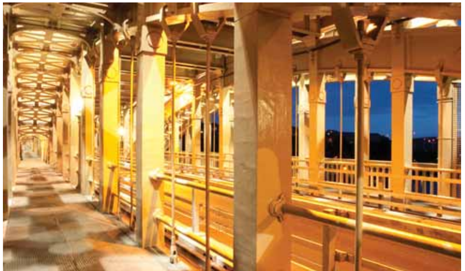
High Level Bridge, NewcastleGateshead
