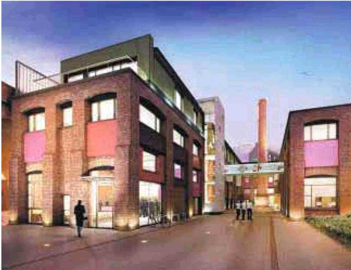
CHANGES How the development will look when the conversion is complete. Below, the Steenbergs Yard now
